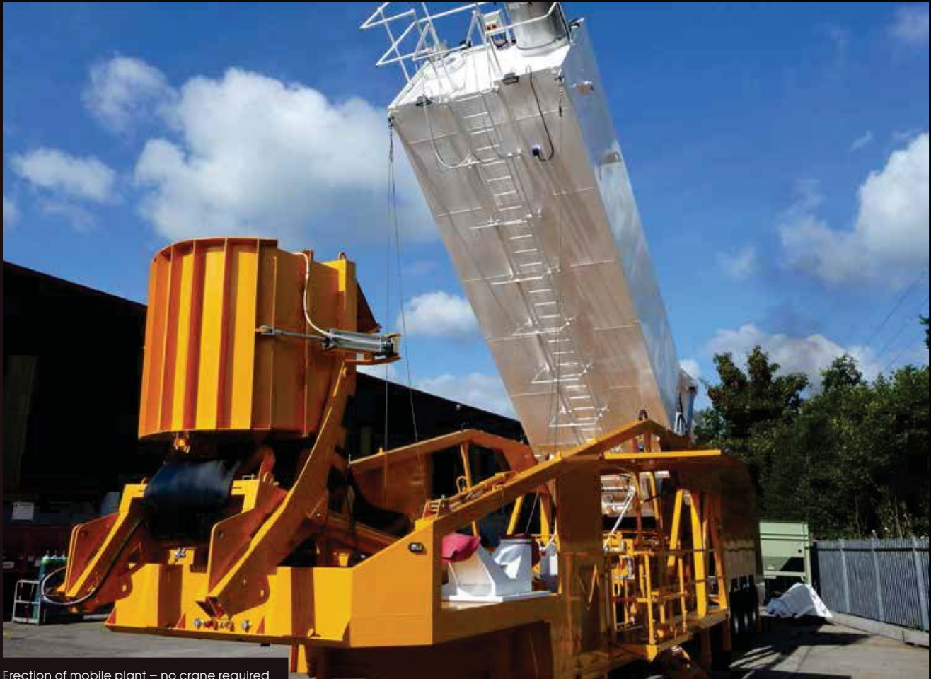
Erection of mobile plant – no crane required
