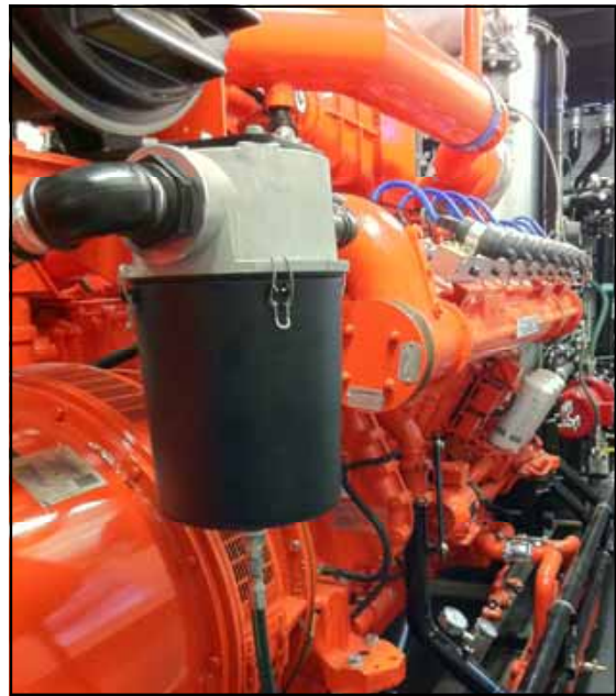
Closed Crankcase Ventilation System Guascor Engine Installation
